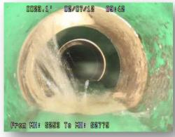
The most common chemical grout used to remotely seal pipe joints, lateral connections and laterals is PR10 acrylamide grout. Having a very low viscosity (1-2 cps), it can easily be pumped through 600-800 feet of hose & small defects that allow groundwater infiltration.
