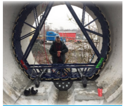
Packer for pipe 96" pipe with cunette
