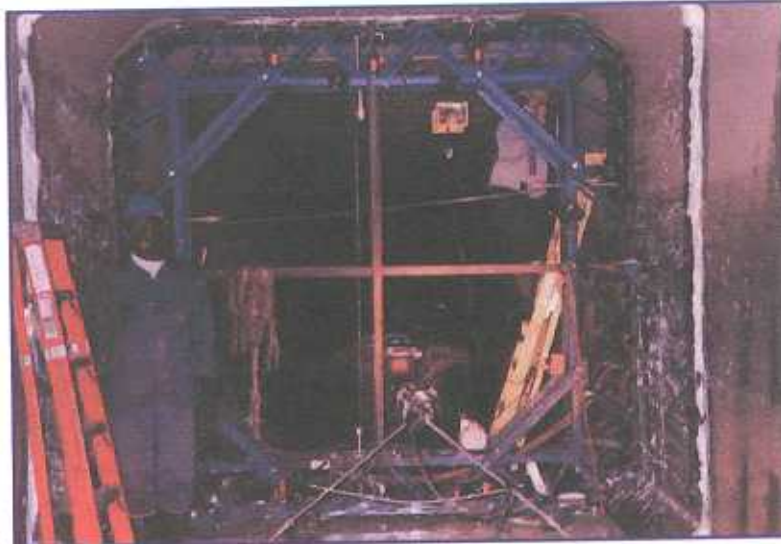
A custom-designed packer grouts and seals the culvert joints.
