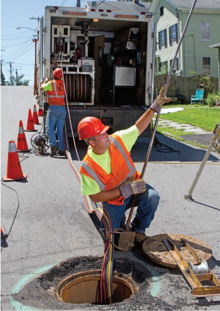
Crew leader Charlie Roberts (foreground) sets the Logiball roller while technician Jason Mahler monitors the status from behind.
