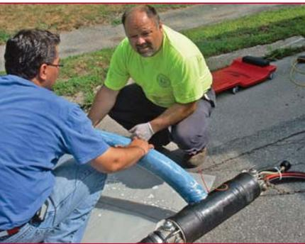
Grout truck operator Gary Millington (in fluorescent safety shirt) helps Marc Ancil of Logiball lubricate the inflated bladder with silicone. After lubrication, vacuum will retract the bladder into the hose carrier.
