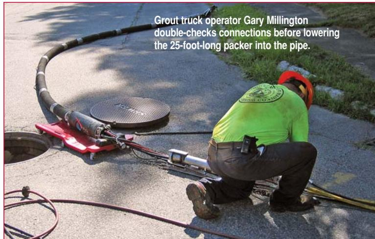
Grout truck operator Gary Millington double-checks connections before lowering the 25-foot-long packer into the pipe.
