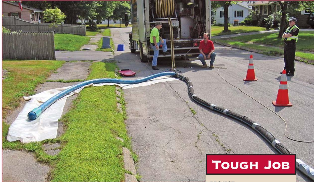
The inflated blue bladder is lubricated and ready for retraction by vacuum back into the hose carrier.
