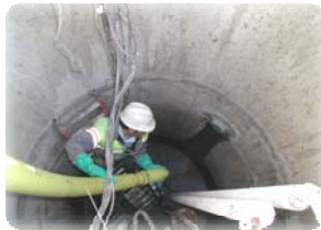
Man entry packer with lateral plug to grout 27" long in a 6" lateral.
