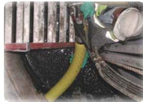
Man entry packer with lateral plug to grout 27" long in a 6" lateral.
