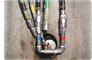
Man entry packer with lateral plug to grout 27" long in a 6" lateral.
