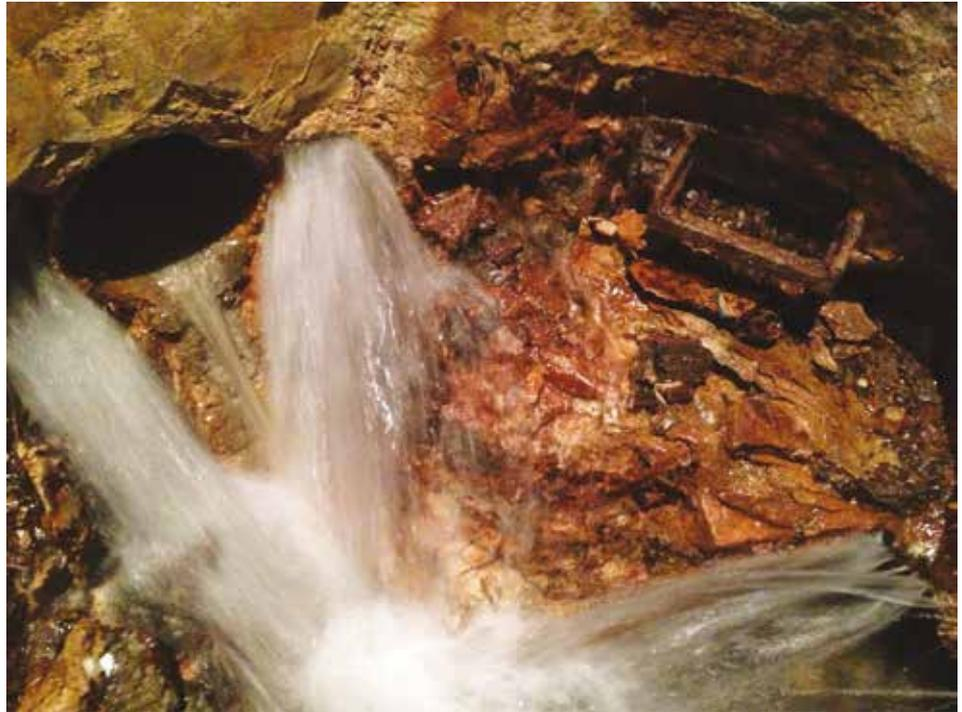
**Groundwater infiltration through cracks in a manhole.**
