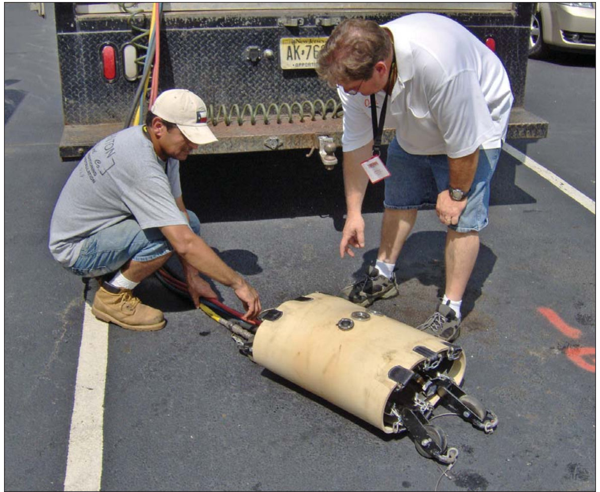
Antonio Rocha (left) from Oswald Enterprises Inc. in Belford, N.J., attaches hoses that deliver air and grout to the 14- by 23-inch elliptical packer custom-built by Logiball Inc. Project manager John Read oversees the process. (Photo courtesy of Oswald Enterprises Inc.)
