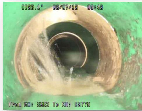
The most common chemical grout used to remotely seal pipe joints, lateral connections and laterals is acrylamide. Having a very low viscosity (1-2 cps), PR 10 acrylamide grout can easily be pumped through 600-800 feet of hose & small defects that allow groundwater infiltration.
