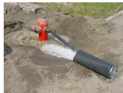
Hydrant Flow Diffuser: Keep the flow under control when flushing fire hydrants.
