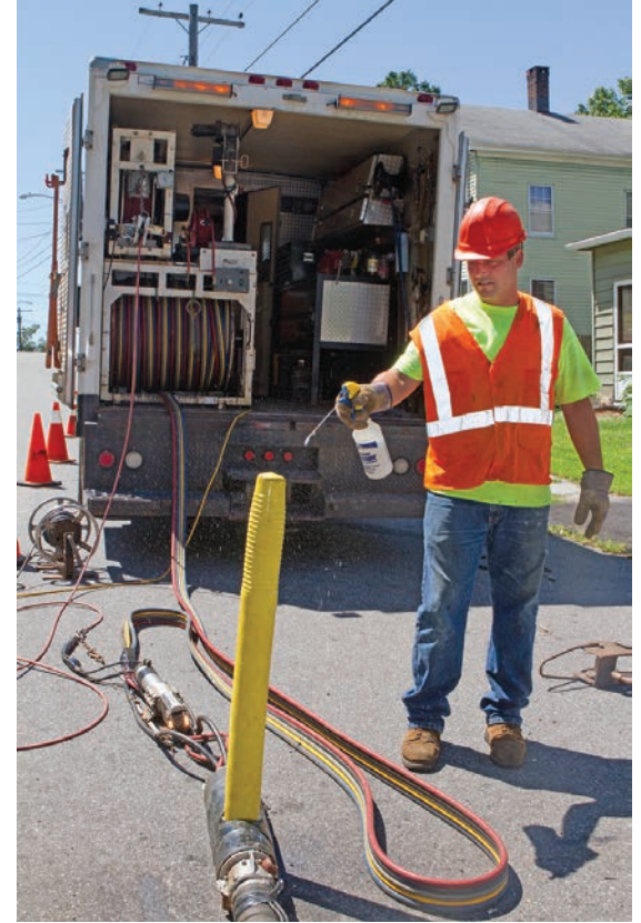
Above: Inside the grout truck, crew leader Charlie Roberts operates Logiball, CUES and Aries equipment, testing and sealing individual laterals. Right: Technician Jason Mahler lubricates the service bladder for the Logiball lateral sealing equipment.
