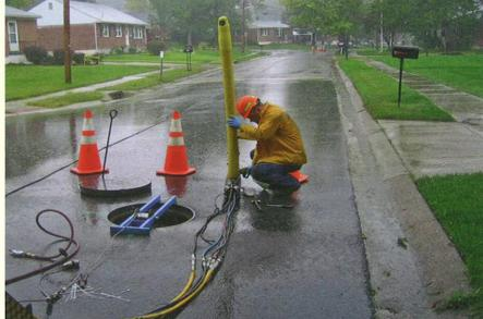
Magill said acrylamide gels are the most widely used chemical grout for lateral repairs. Others are acrylic gels, acrylates and
