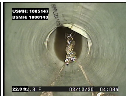
Photo at the bend A few minor wrinkles at the Top were expected
