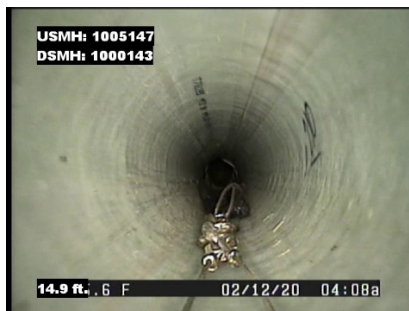
Photo dropping into siphon
