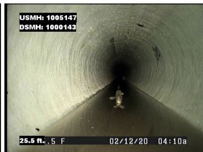
Photo in the main horizontal main barrel section of the siphon
