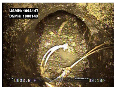
This is right where the siphon starts its horizontal run
