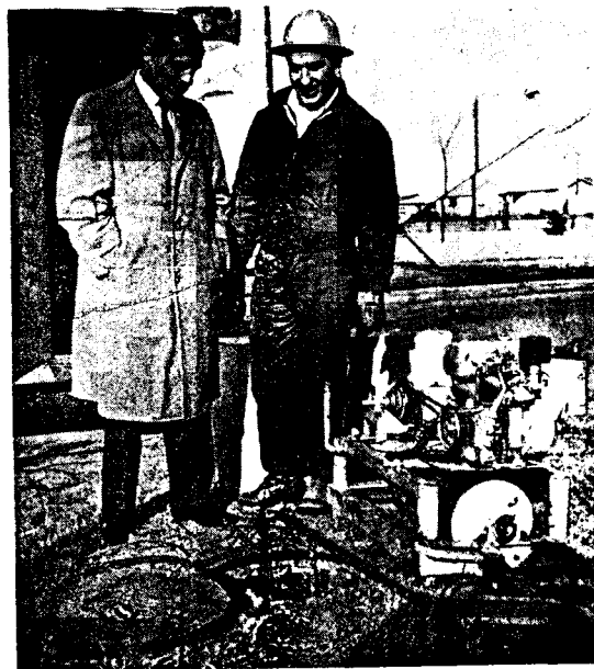
The camera drops into a manhole and starts its journey.
