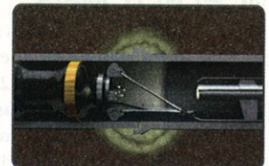
Grout collar stops infiltration
