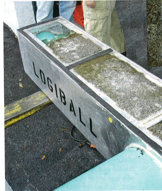
Above-ground demonstration where the chemical grout seals the voids between the backfill materials around the service connection and 20 in. and up
