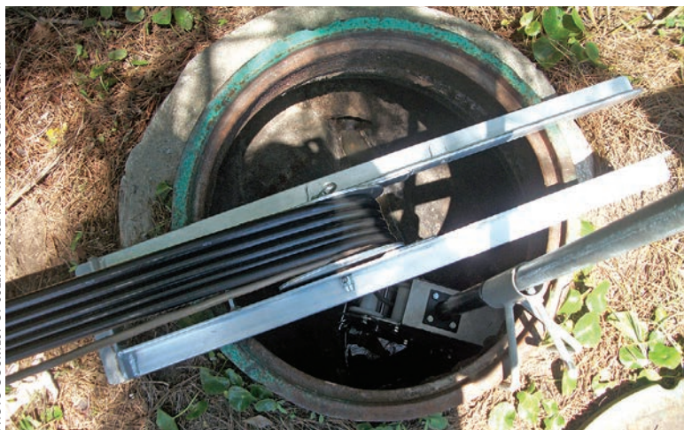
A camera cable, hoses carrying the two-part grout mix, and air lines for the grout packer pass over a roller on a manhole. The grout packer is attached in the sewer line.
