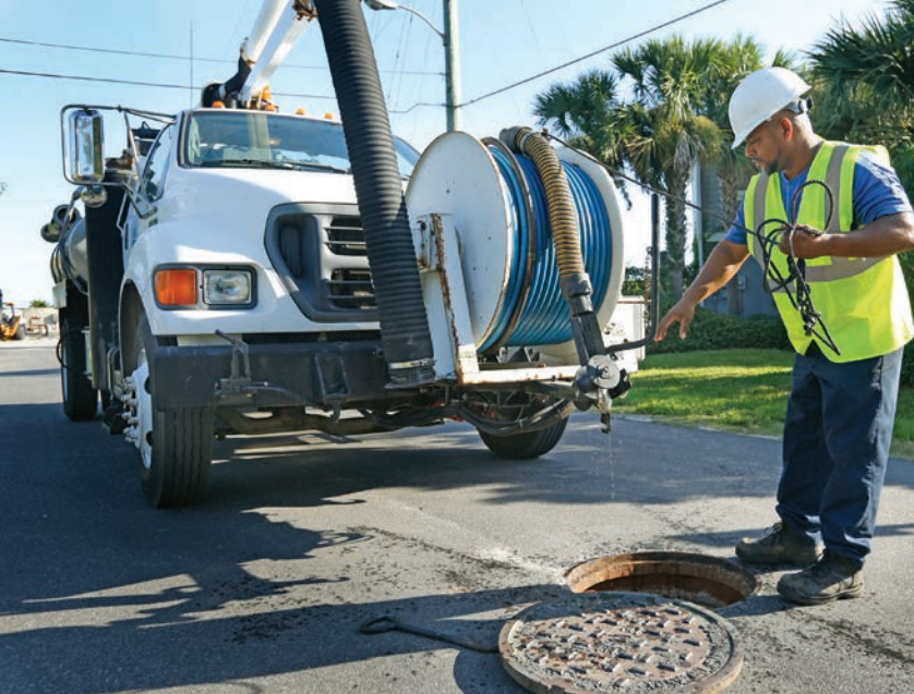
Darrell Noisette wraps up after cleaning a sewer main.
