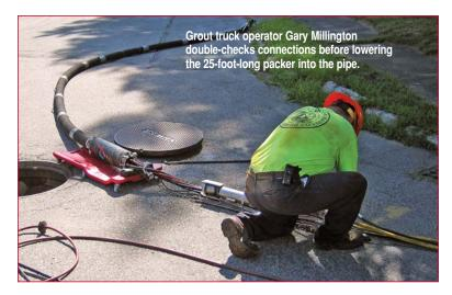
annular space. Grout flows through this passage, out the bad joints, and gels with the surrounding soil. Millington could see water running as the bladder approached the joint, and stop after the grout was injected. The average annular space held 12 gallons of grout. The most used in any repair was 26 gallons. Pressure monitoring told Millington when laterals were sealed.
