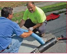
Grout truck operator Gary Millington (in fluorescent safety shirt) helps Marc Anctil of Logiball lubricate the inflated bladder with silicone. After lubrication, vacuum will retract the bladder into the hose carrier.
