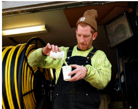
Figure 3 – Checking Gel Time
