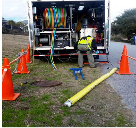
Figure 9 – Long Sock Fracture Grouting
