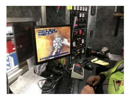
Working from opposite sides of the pipe run, Michels lining crews installed pressure pipe from pits three and four while Michels grouting crews tested and sealed using the latitudinal flexible packer from pits one and two.
